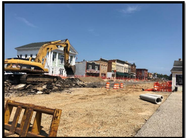
Davis Construction worked to remove all the pavement and sidewalk from Gremps Street to Kalamazoo Street
