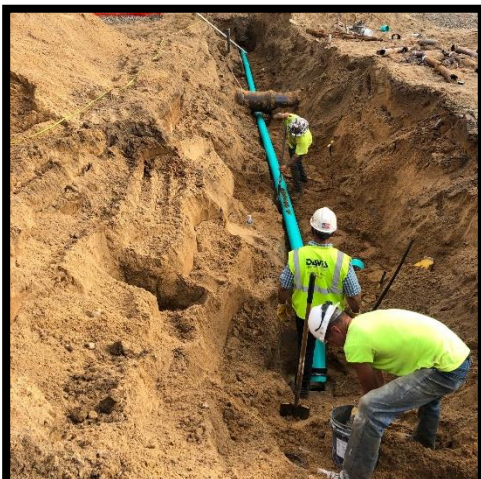
Davis Construction placed new sanitary laterals this week
