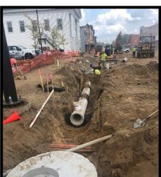
Underground construction was completed in the 100 block of E. Michigan Avenue with the installation of the final storm sewer in the area.
