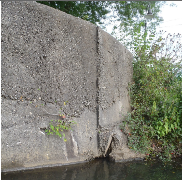
Photo 10 Left Spill Tube Structure, downstream asphalt overlay
