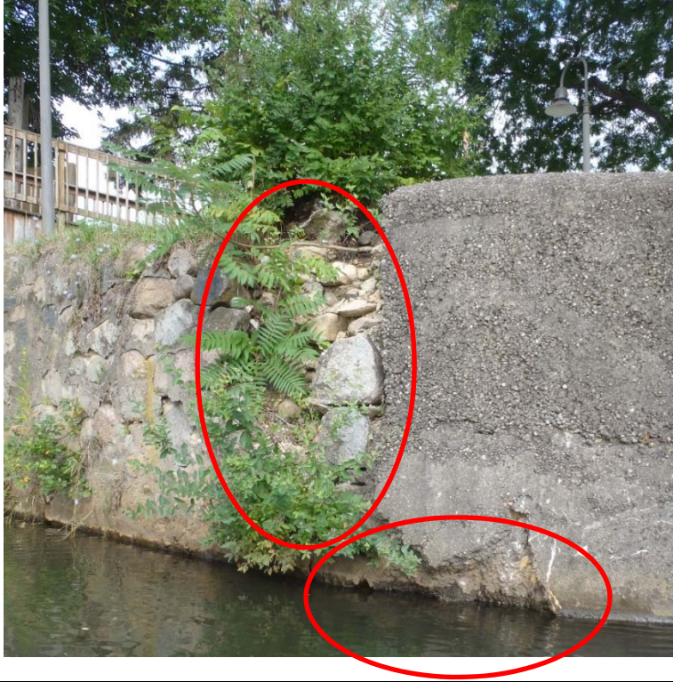
Photo 11 Left Spill Tube Structure, downstream wall deterioration
