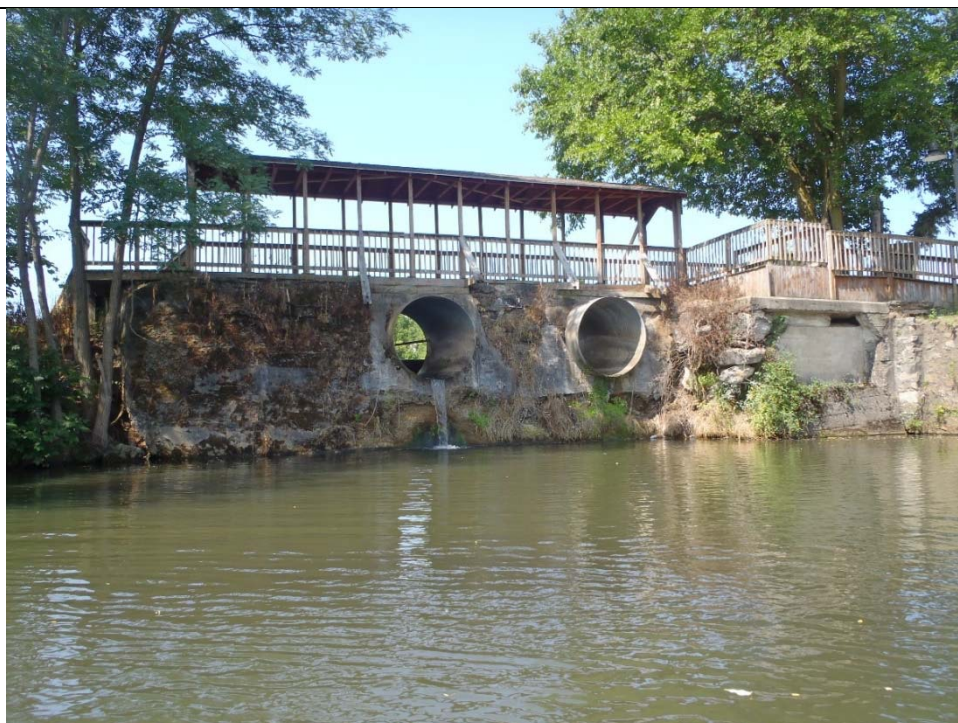
Photo 2 Spill Tube Structure, downstream
