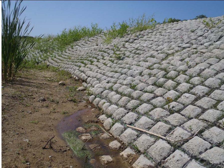
Photo 9 Seepage on Downstream side of Emergency Spillway
