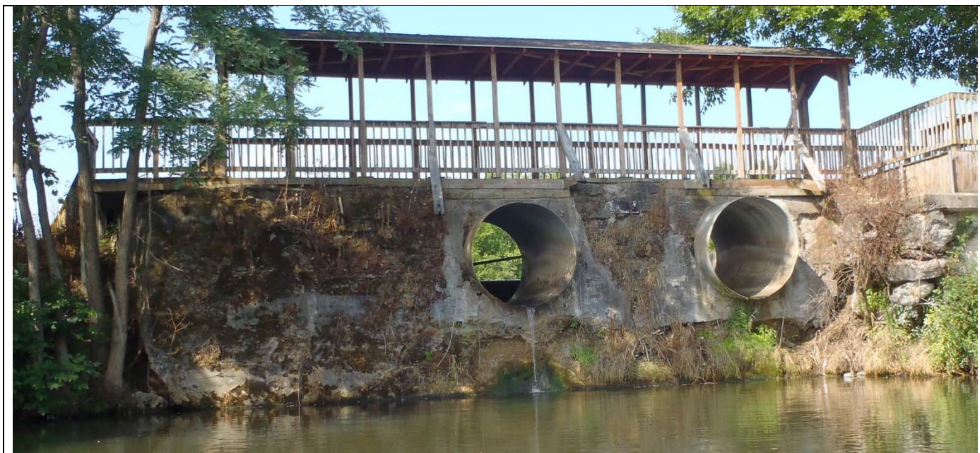
Photo 15 Spill Tube Structure, downstream
