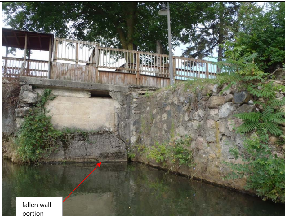
Photo 12 Left Spill Tube Structure, downstream wall and box structure
