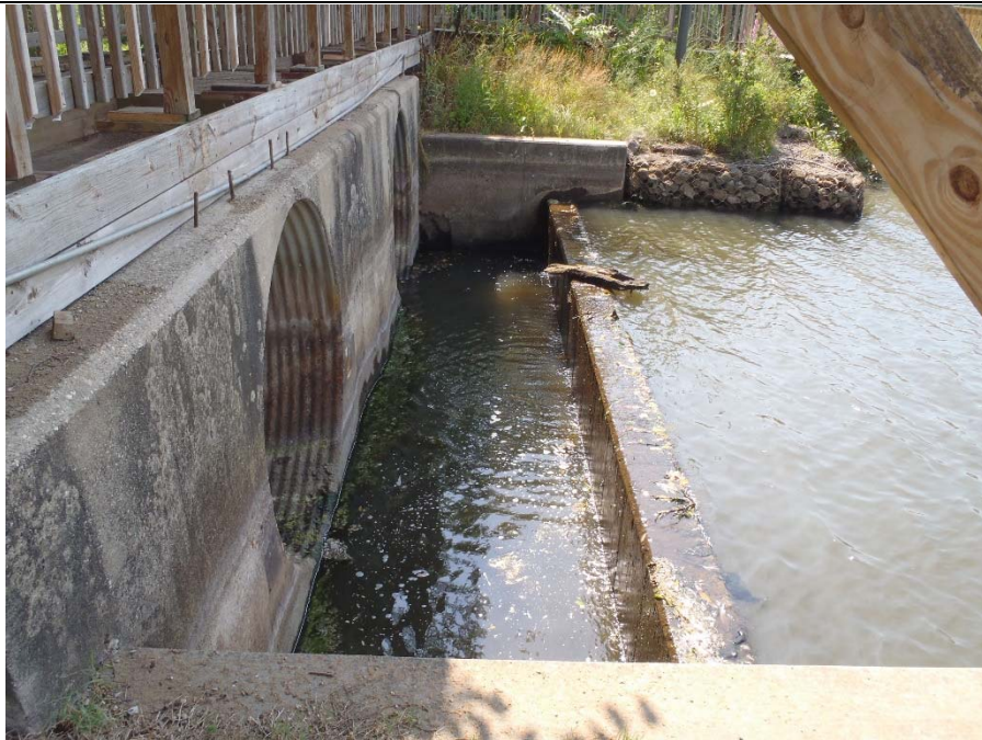
Photo 18 Upstream Spill Tube Structure Weir
